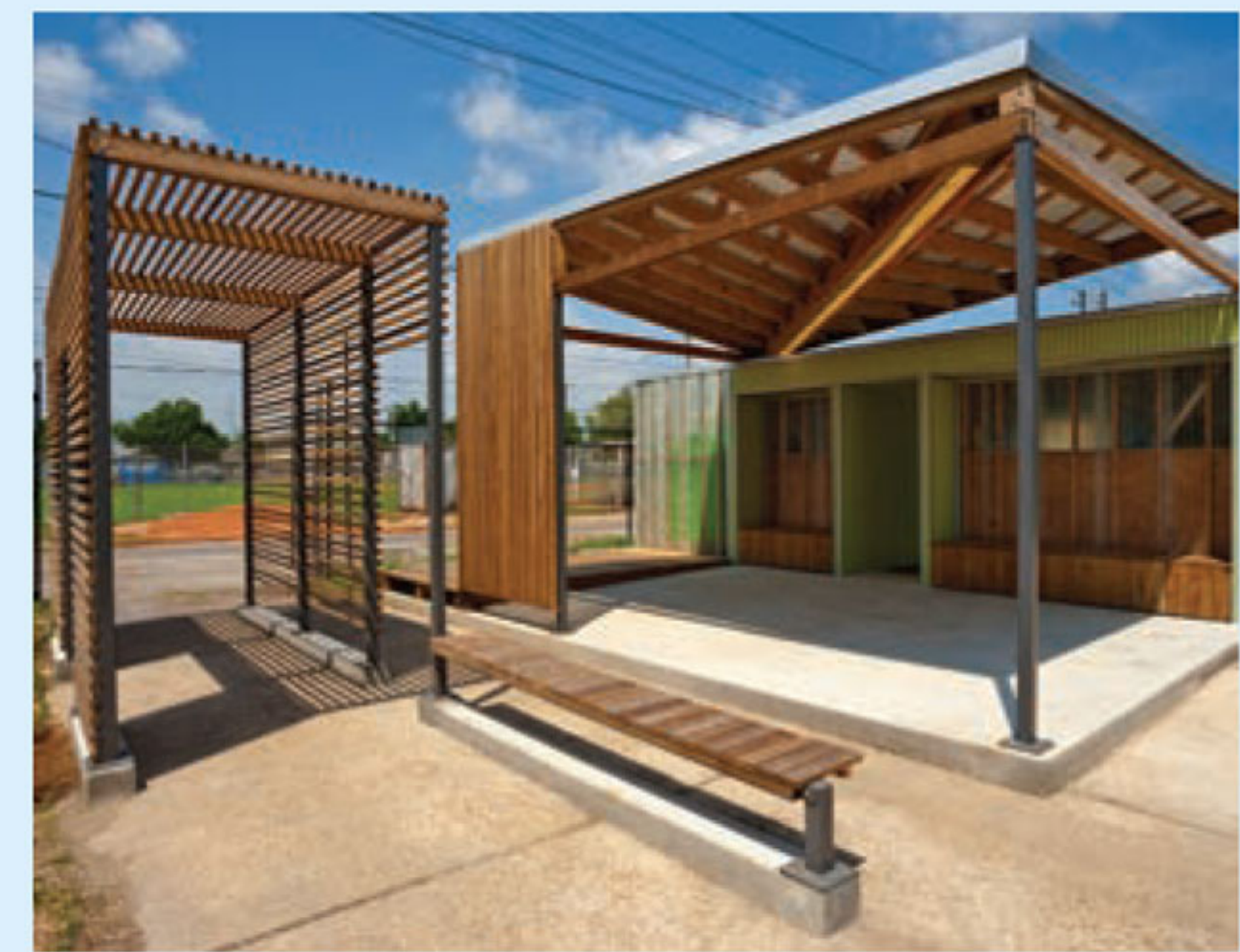
A pavillion at a local green market was designed and built by students through Tulane City Center.
